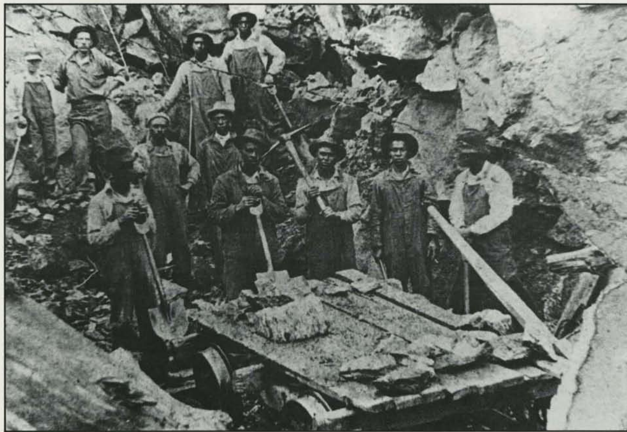
A tremendous amount of manual labor was needed to build roads and railroad beds through the mountains. This crew worked in the Wise County area, date unknown. (Courtesy Susie Baker)
