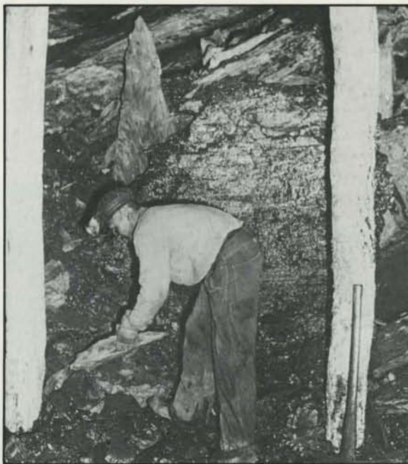
A black miner separates slate from coal in an unidentified mine. (Courtesy Grubb Photo)
